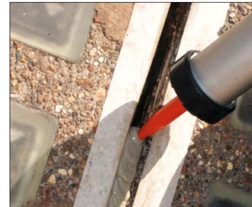
3. We can seal cable, pipe openings and construction joints using high performance sealants
