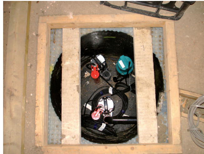
Two mains powered pumps were installed to the sump.
