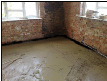
New concrete slab being poured
