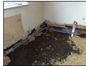
Hardcore being laid.
