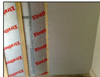
Battens & plasterboard added
